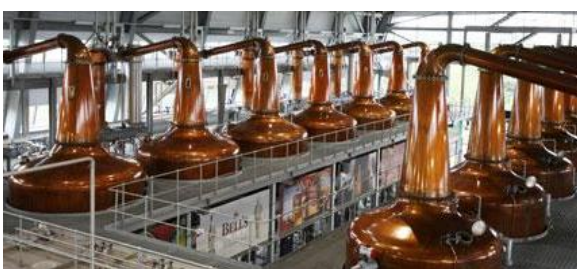
The Roseisle Distillery is the first new large-scale distillery in Scotland for over 30 years. It combines the best of modern and traditional techniques to produce quality spirit for brands including Johnnie Walker and Buchanan's.
